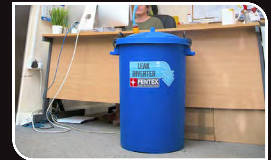
Drains into Reservoir Drum
