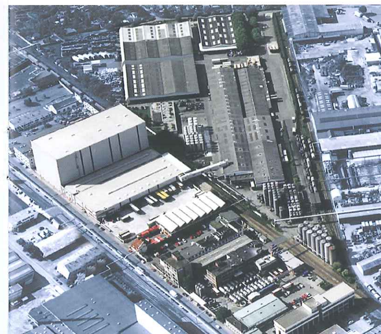
FUCHS EUROPE SCHMIERSTOFFE plant in Mannheim/Germany
